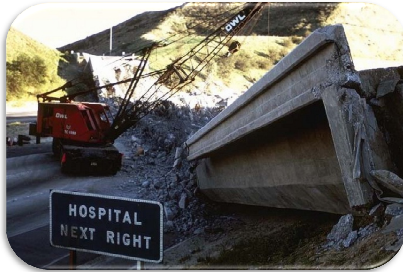
Figure 1.1: Collapsed bridge resulting from the 1971 San Fernando earthquake (DesRoches, 2012)
