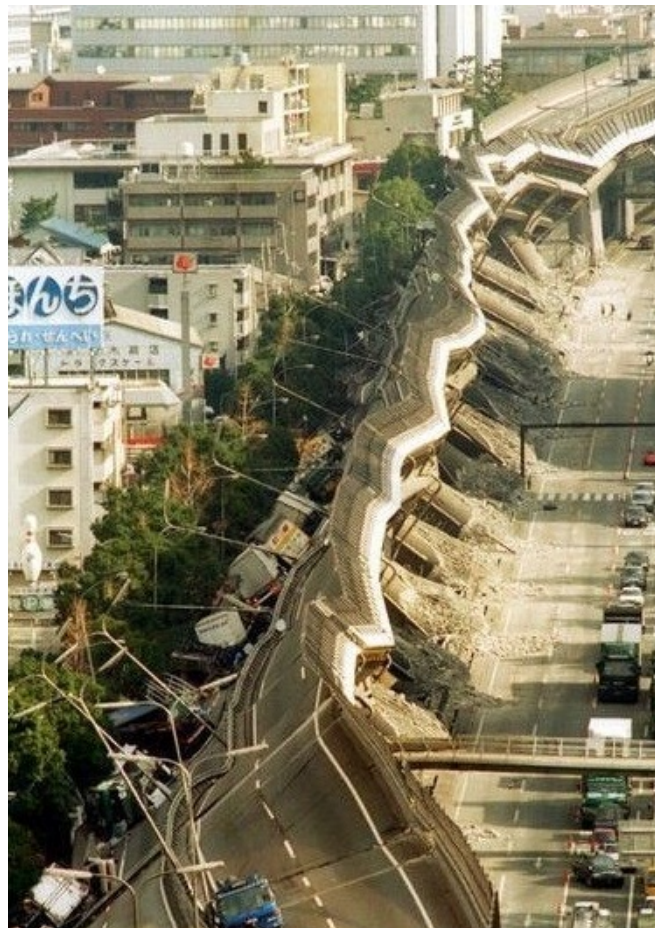
Figure 1.2: The collapse of the Hanshin expressway in the Kobe earthquake (Johansson, 2000)
