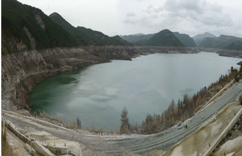
Photograph 4: Itoiz Reservoir completed (2008)
