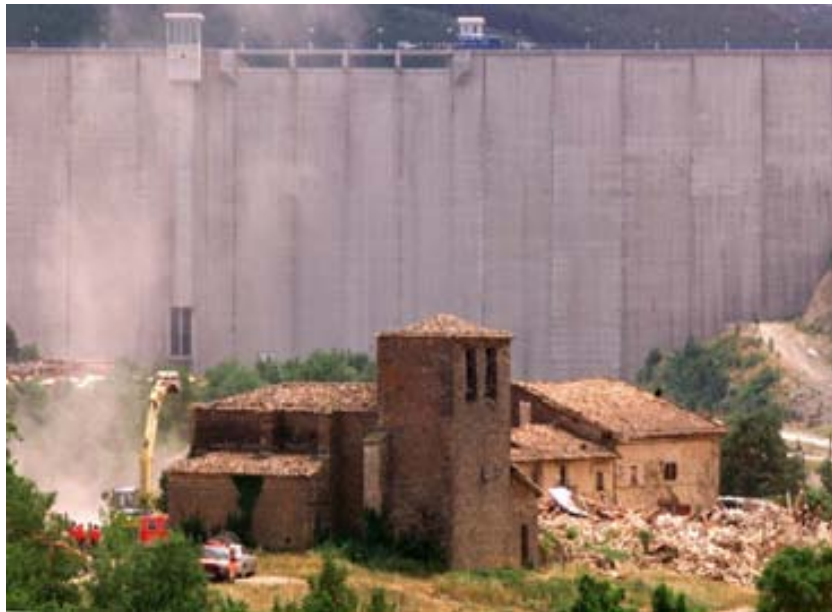
Photograph 6: Demolishing starts in Itoiz
