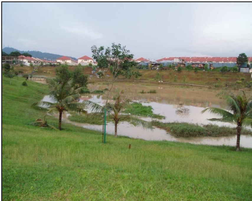
Figure 1.7: Condition of Dry Detention Pond after Storm Event
