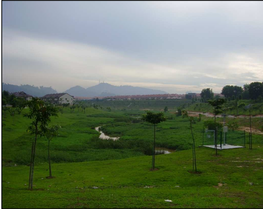
Figure 1.6: Condition of Dry Detention Pond during Dry Season
