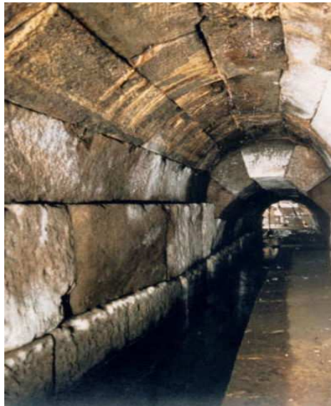
Figure 2.4: View of the Interior of the Cloaca Maxima (Wikipedia, 2008)
