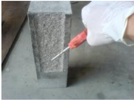
Figure 5: Surface cleansing to remove dust using air compressor
