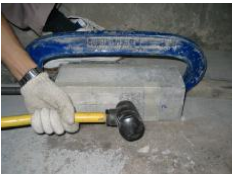
Figure 3: Hacking with air tool hammer
