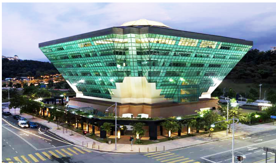
Figure 1.3: Diamond Building, the eight-story Green Building in Putrajaya Malaysia. Source: Lim Japheth (2013)
