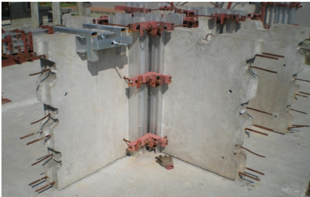
Figure 1.5 Innovated modular moulds for wet-joint grouting at site
