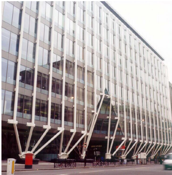
Figure 1.3 Fleet Place House (London, UK)
