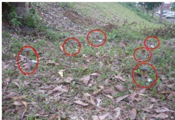
Figure-1. Tensiometer installed at toe of slope.
