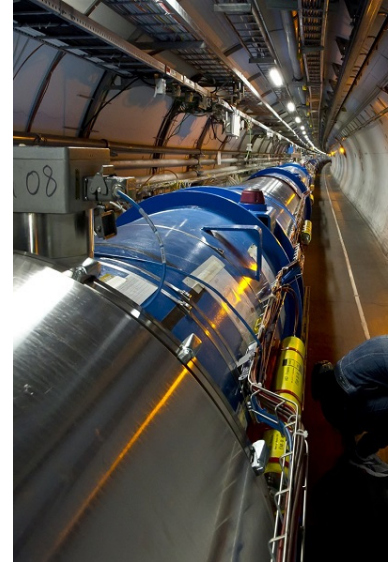
The LHC tunnel. Adapted from [183].
