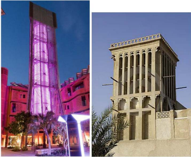
Figure 8: The 45 m tall wind tower in Masdar city - capturing upper-level winds and directing them to the open-air public square at its base
