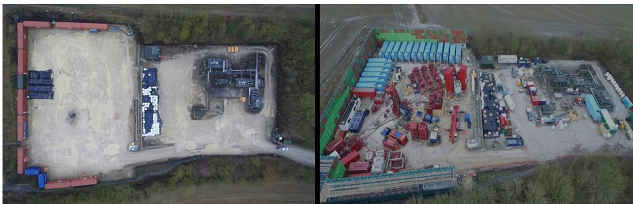
Fig. 6. Images of the Third Energy Kirby Misperton well site in December 2017 (left hand side) and April 2018 (right hand side), illustrating the extra equipment brought onto the site in preparation for shale gas extraction. (Credit: Eddie Thornton).
