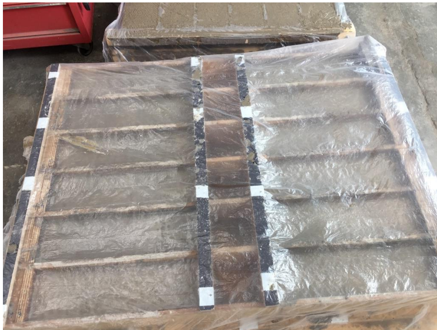
Figure C. 1 Substrate concrete casting
