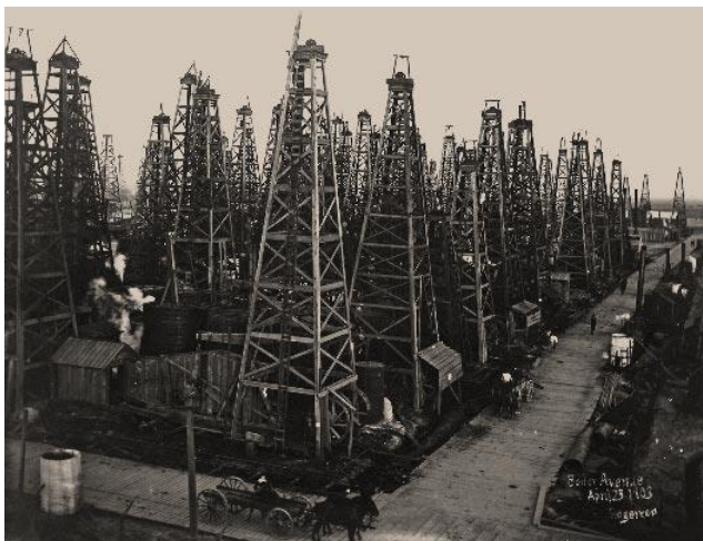
Figure 2: Boiler Avenue at Spindletop*
