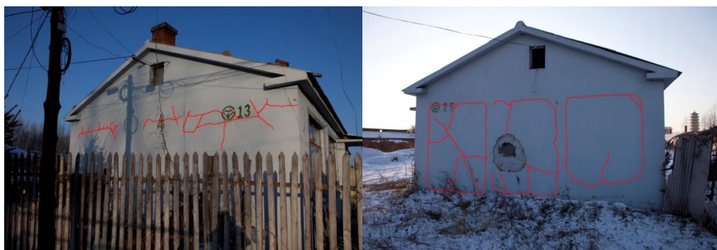
526 Figure 13. Cracks (highlighted in red) on surface of brick frames (left) and between 527 straw bales and frames (right).
