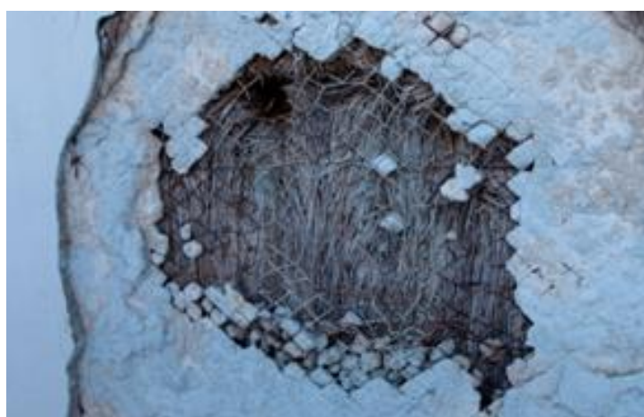
530 Figure 14. Straw degradation in the gable end of a non-resided straw bale house 531 in ADRA project.
