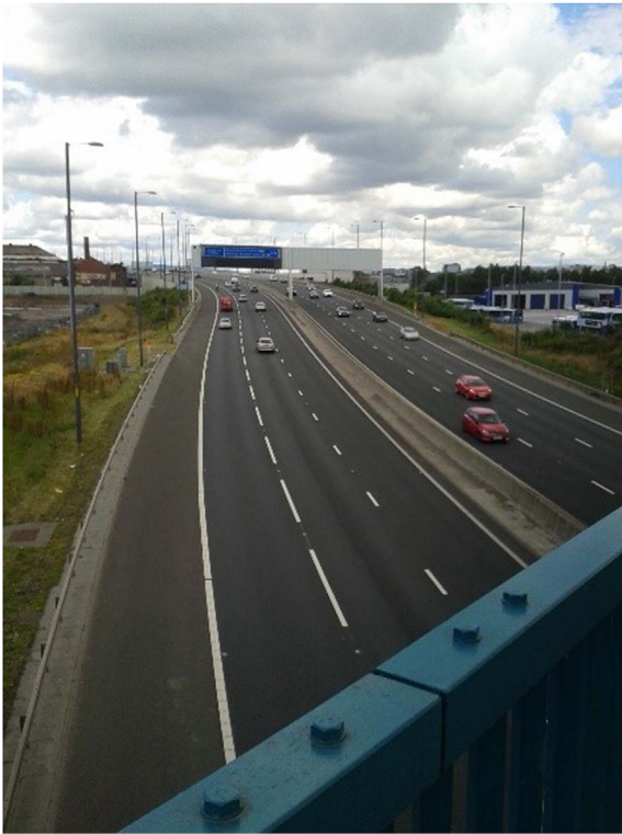
Fig. 2. M74 extension passing beneath an existing street in Govanhill, Photograph © study participant and reproduced with permission.
