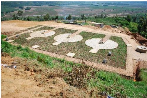
Figure 3 : 3x100m<sup>3</sup> digesters, built during phase 3 of construction, due to the increasing number of inmates in the prison.
