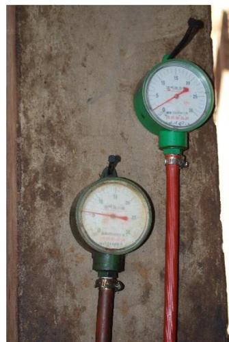
Figure 4 : manometer, used to measure biogas pressure. According to the person in charge, the outlet pressure can reach 15 to 16 kPa
