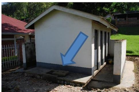
Figure 1: latrine, including human waste collector (blue arrow)
