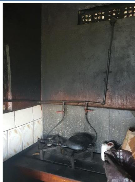
*Figure 1: biogas pipes, where two stoves are still connected but not currently in use. A manometer is visible up right.*
