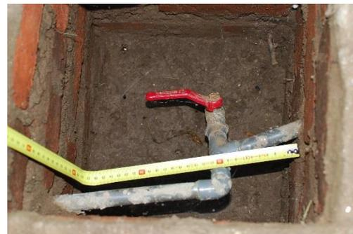
*Figure 4: purge valve that should be open every day at least few seconds.*
