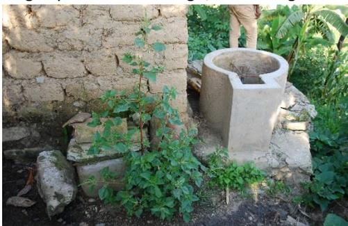
Figure 1: feed chamber (for cow dung) (right) and entrance for human waste to the digestion chamber (left).
