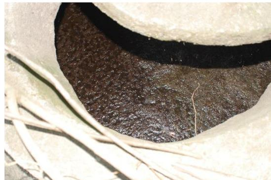
Figure 3: slurry in evacuation chamber (and probably digestion chamber) that should be removed before rehabilitation.
