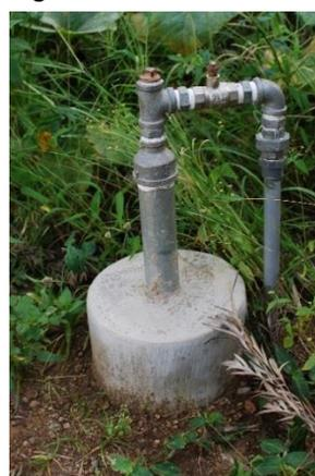
Figure 2: biogas exit from digestion chamber.
