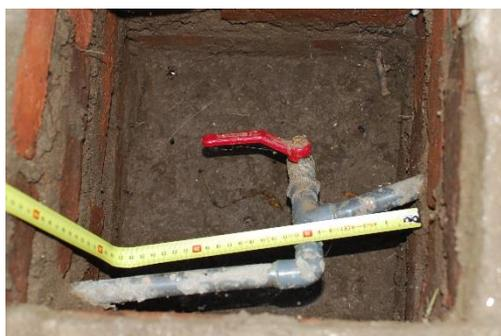
Figure 1: biogas tap, allowing the evacuation of condensated water in pipes.
