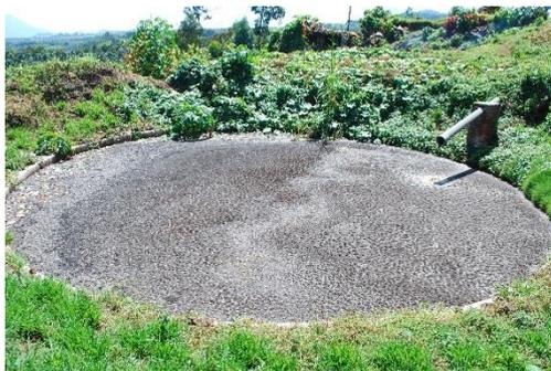
Figure 3: retention pond, containing slurry evacuated from 4x100m<sup>3</sup> digester (diameter 7m, depth 1.5m).
