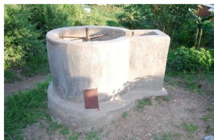
Figure 2: feed chamber, where cow dung is stirred.
