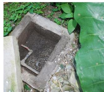
Figure 4: condensate tab to remove water from gas pipes.
