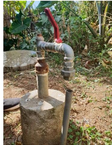
*Figure 3: gas tap should be carefully controlled, due to the several joints on it.*
