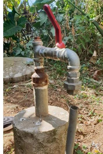
*Fig.2: dome outlet valve. Only a small amount of biogas was exhausted when it was opened.*
