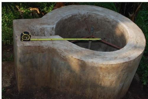
Figure 1: feed chamber, including scale (50cm).
