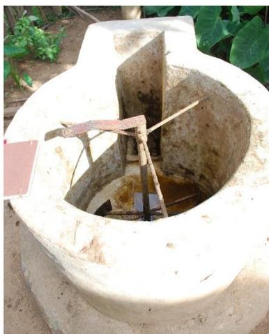
Figure 1: feed chamber, where feed is added every 2 days. Stirring is used to mix the feed before it enters the digester.
