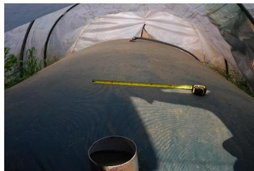
Figure 2: internal view of plastic bag digester.
