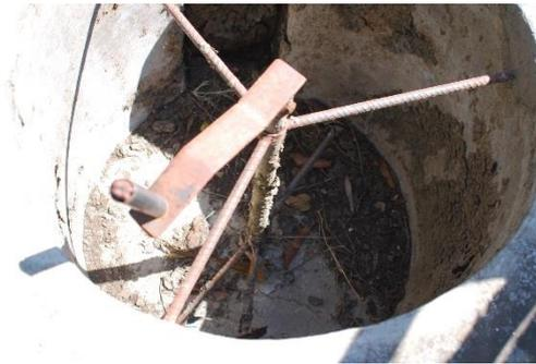
Figure 2: stirring equipment where rust should be removed before rehabilitation.
