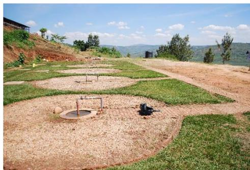
Figure 1 : 4x100m<sup>3</sup> digesters, built during phase 1 of construction.
