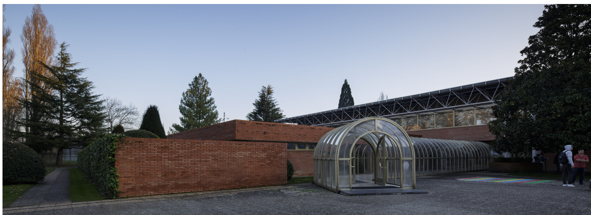
Figure 3. Office building, School of Architecture (University of Navarra).
