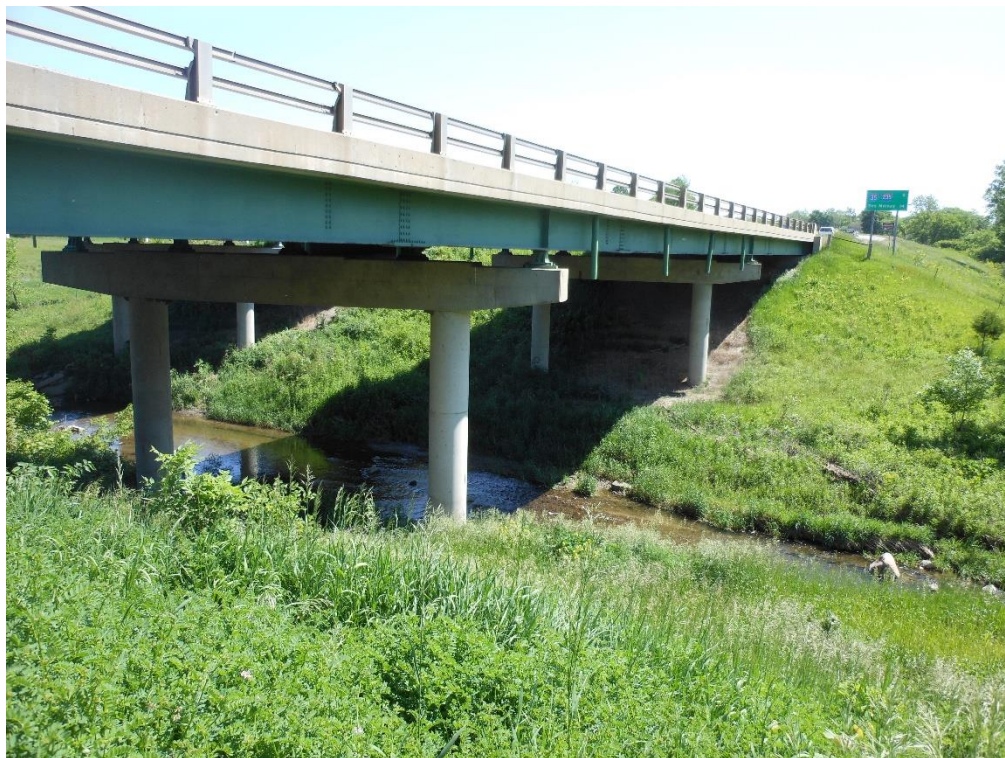
Figure 3.2. Demonstration bridge FHWA #22380 on Interstate 80
