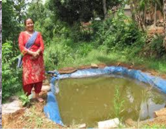
Figure 6. Rainwater collection plastic pond
