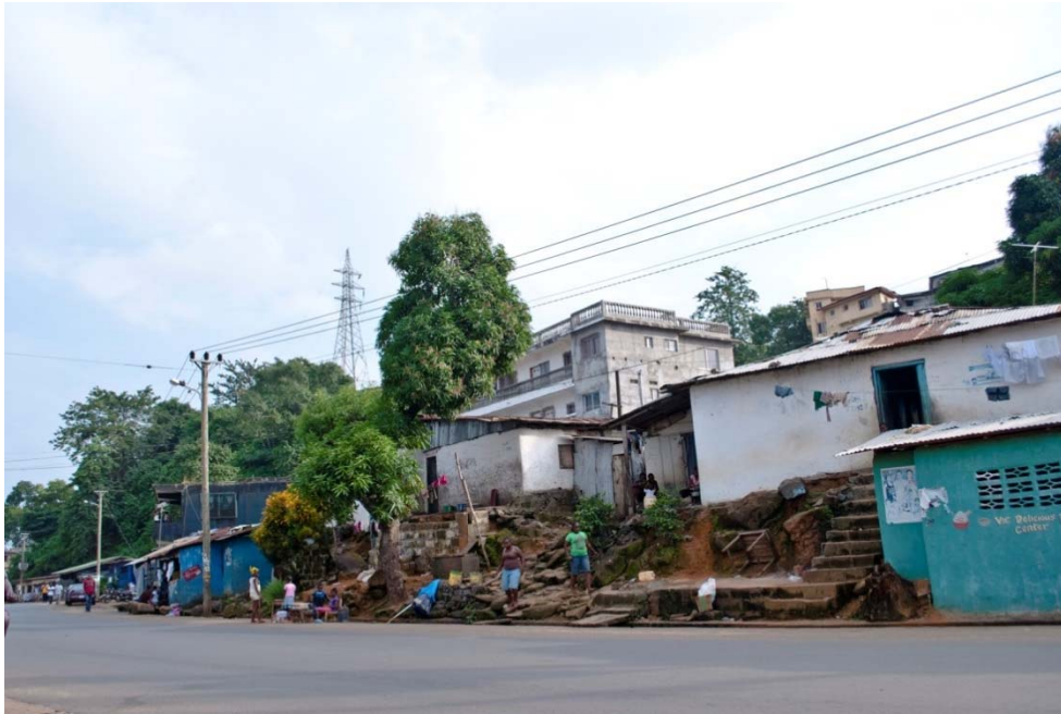
Figure 14: Jallah Town Road, looking west at the "established" section of the community.
