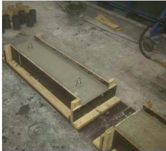
Figure B. 1: Casting of the reinforced concrete slabs and specimen
