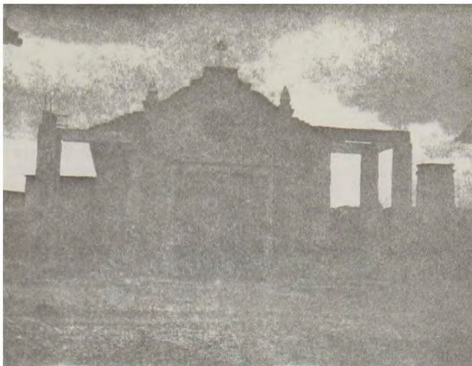
PHOTOGRAPH: IV CHURCH BUILT WITH AIDS PROVIDED BY MIGRANTS OF C.S.D.M.
