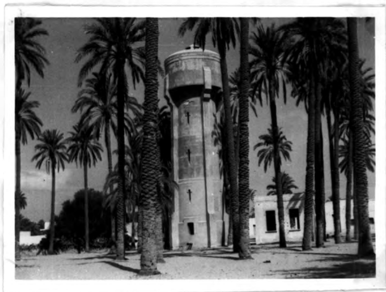
The main water reservoir in Zavla
