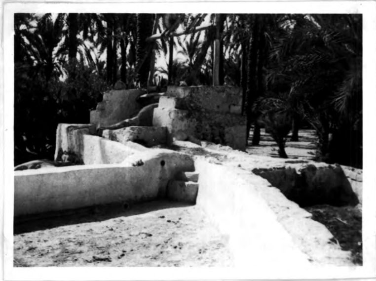
A typical well with two storage tanks, Zavia.
