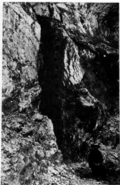
An exposed shaft at Rio Tinto, Spain, showing the footholds.
