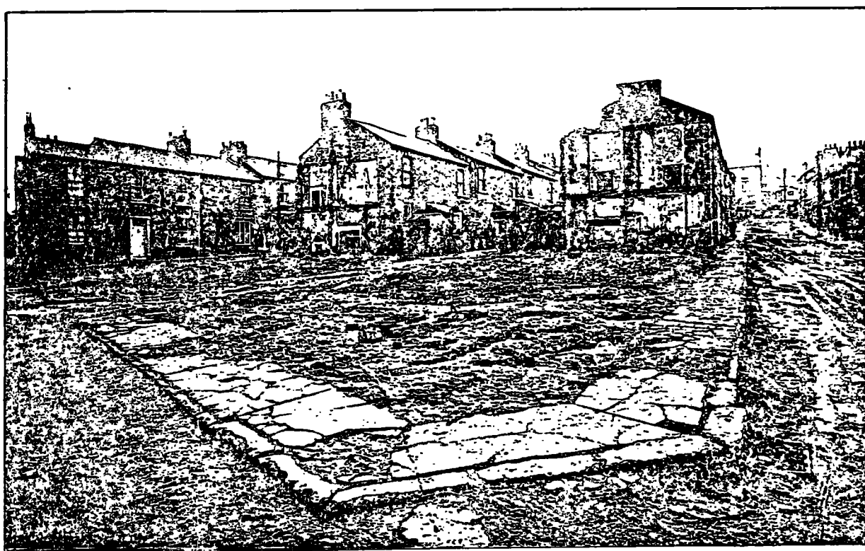
"Bulldozers gnaw away at the end houses and the village is slowly eaten away" Daily Telegraph Magazine, 1969
