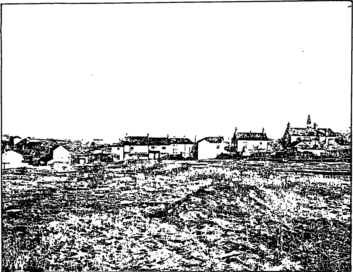
Witton Park, 1979 View facing Main Street across the demolished housing sites.
