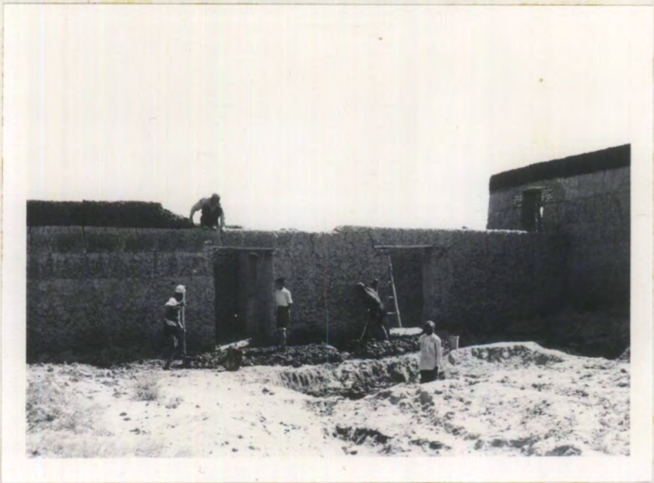
Haji Nasir - wall being constructed in courses by a party of village workmen.
