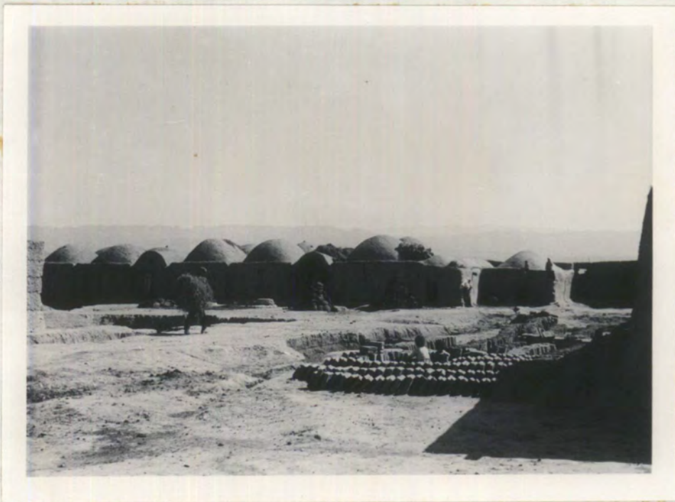
Haji Nasir - mud bricks outside the house of the builder in the village.
