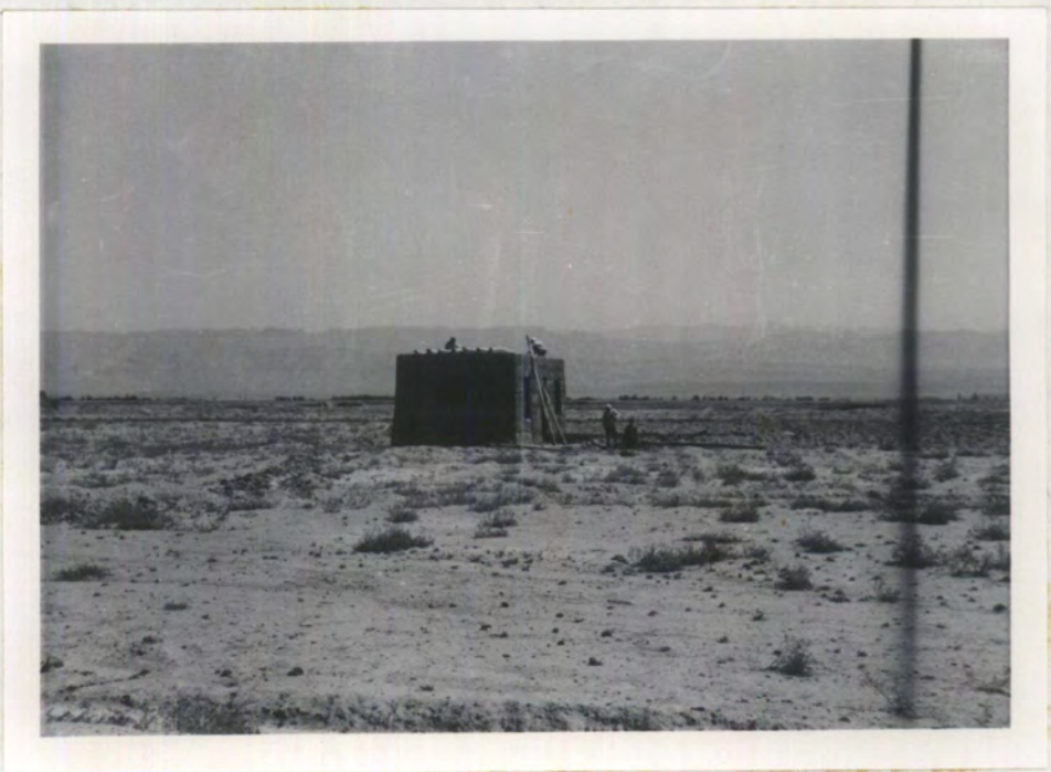
Haji Nasir - poles being laid on house walls before roofing with mud.
