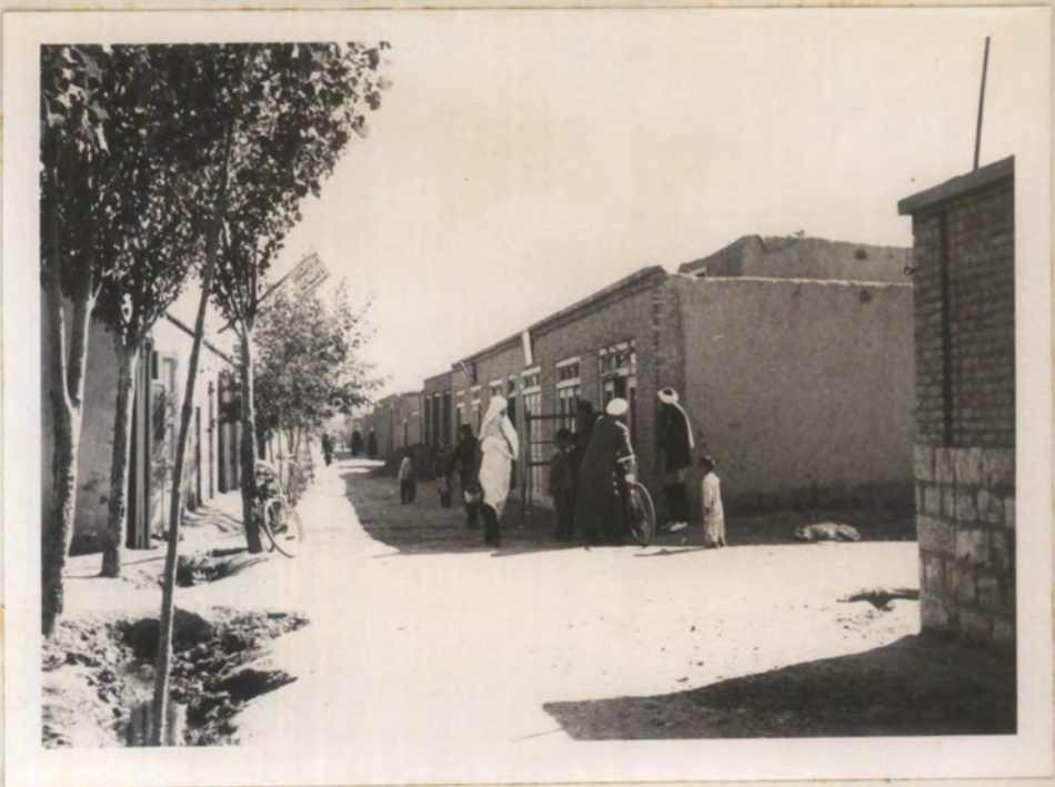
Haji Nasir - street of shops in the new settlement.
