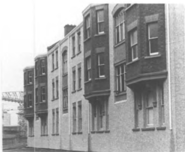
ILLUSTRATION 2-22 Harrison Buildings, Silver Street, Sunderland; opened in 1903 and photographed in 1976 during renovation.
