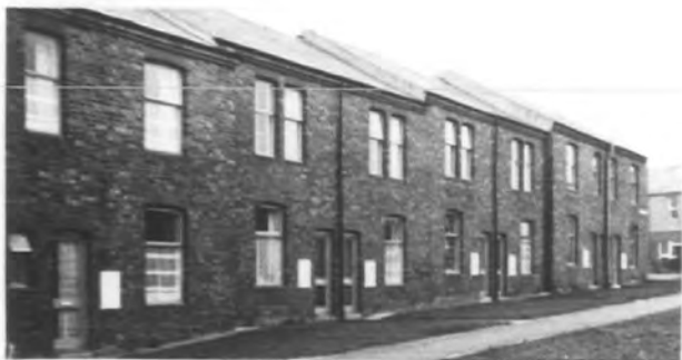
ILLUSTRATION 2-25 House Terrace, Usworth. These rather plain terraced council houses have recently been modernised.
