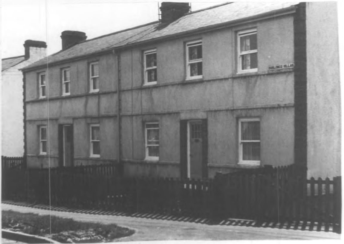
ILLUSTRATION 4-4 Dorlonco Villas, Meadowfield. This second example from the Addison Act stock of Brandon UDC shows a pair of the ill-fated steel and concrete houses assembled from kits supplied by Dorman Long & Co.
