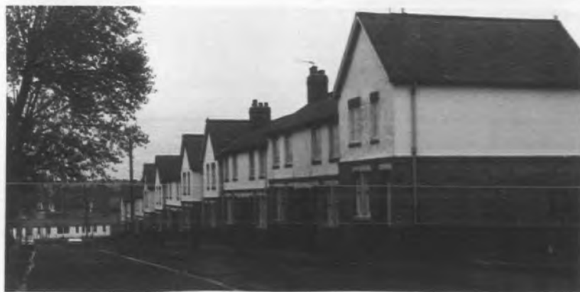
ILLUSTRATION 2-28 Bede Terrace, Chester-le-Street. More imaginative treatment of design is apparent in these somewhat later 1890 Act houses. Note the arched passageways for access to coalhouses and bins.
