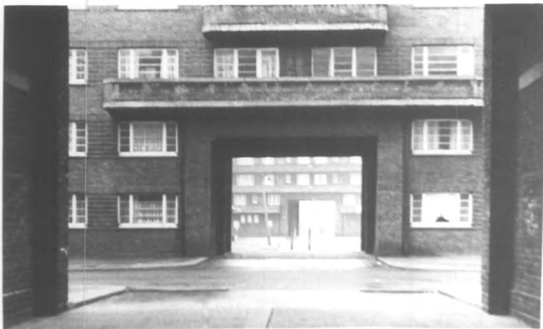
ILLUSTRATION 5-7 The Garths, Sunderland. This unhappy illustration of Art Deco gone wrong comes from the stock of the North Eastern Housing Association. It compares very badly with the 1890 Act dwellings which it faces (see Illustration 2-22) and is an early example of public sector building losing sight of the human scale in housing design.
