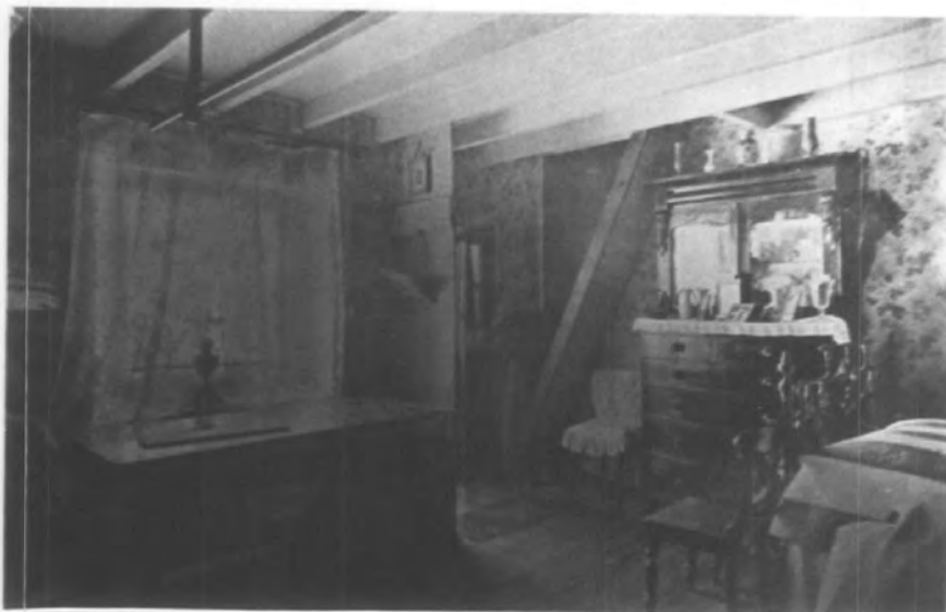
ILLUSTRATION 2-16 Ground floor interior, Marley Hill, c 1907
