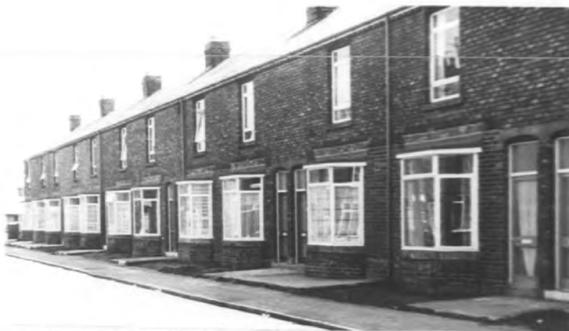
ILLUSTRATION 2-26 North Side Terrace, Trindon Grange. Another fairly plain terrace, completed in 1914, with the addition of bay windows to lend distinction.
