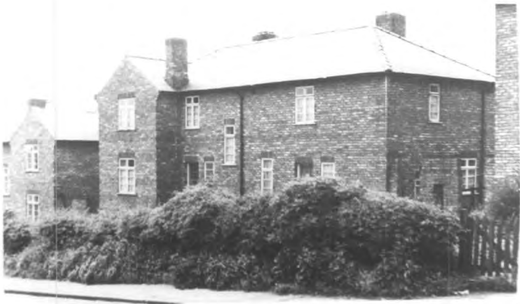
ILLUSTRATION 4-2 Station Road, Esh Winning. The style of these Addison Act houses has a distinct Jacobean flavour - seen in the gables, the unusual fenestration and the tall chimney stacks.
