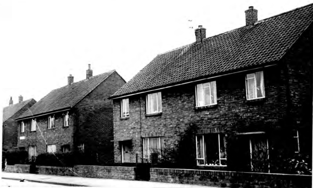
PLATE 4. Shrigley Gardens. In E.D.6. an area of self-contained housing.
