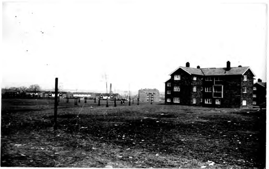
PLATE 18. View across the Park from Kirkwood Drive. Three storey point-block maisonettes flank the Park which, as this Plate shows, is bare and untidy.
