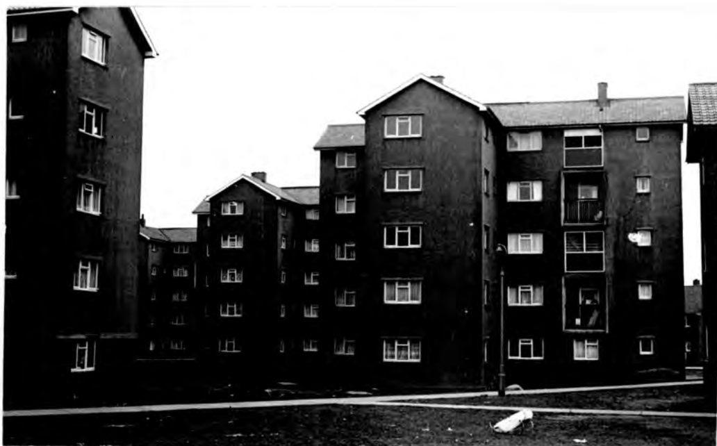
PLATE 11. Five storey point-block maisonettes- Apsley Crescent/Laith Road.
