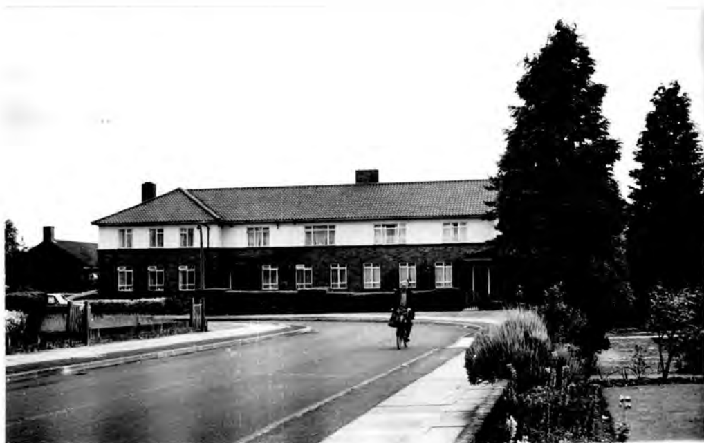
PLATE 44. Two storey flats in Devonshire Avenue.
