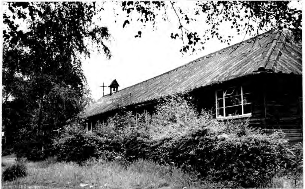
PLATE 55. St. Michael's Anglican Church. Designed as a temporary church in timber.
