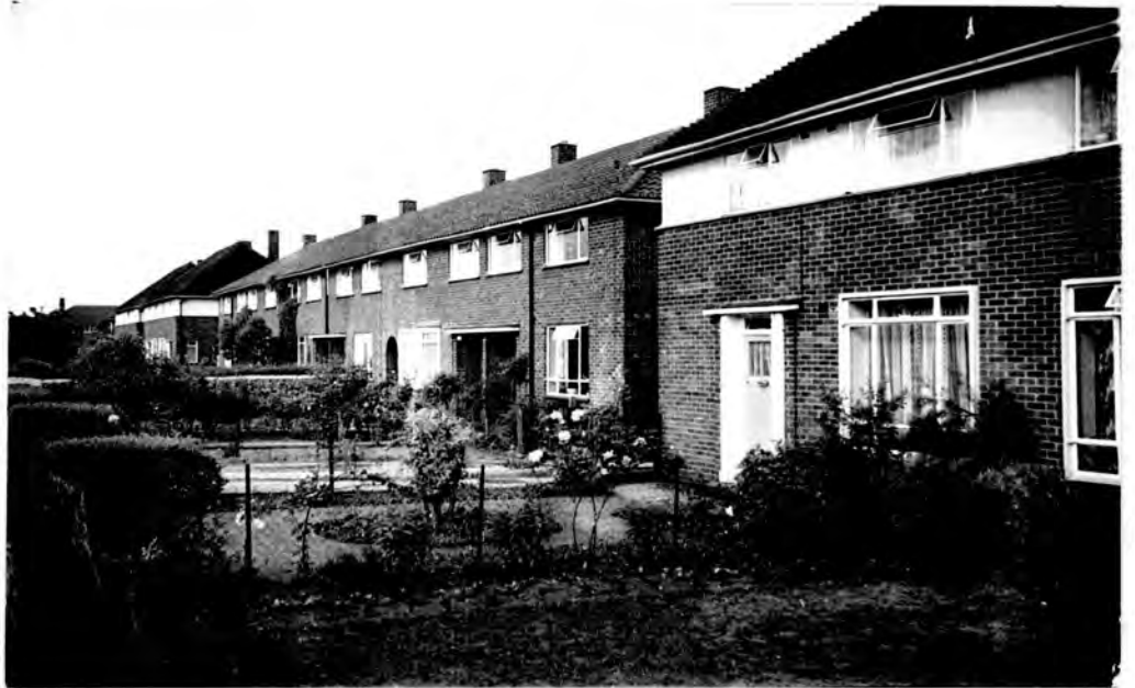
PLATE 35. Self-contained dwellings in Bentham Avenue.
