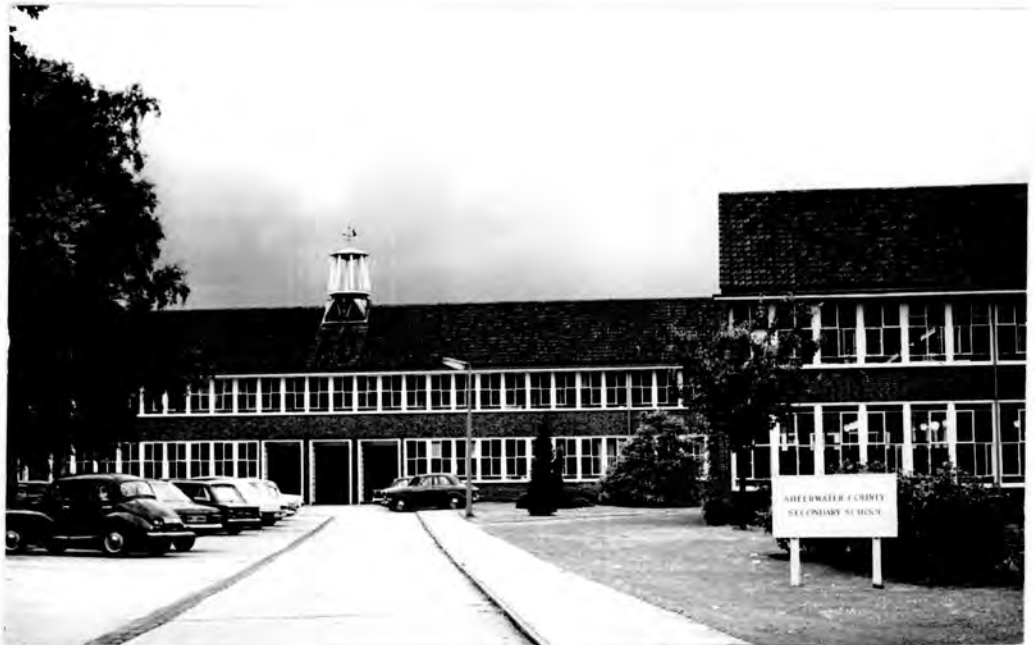
PLATE 51. Sheerwater Secondary School, Albert Drive.
