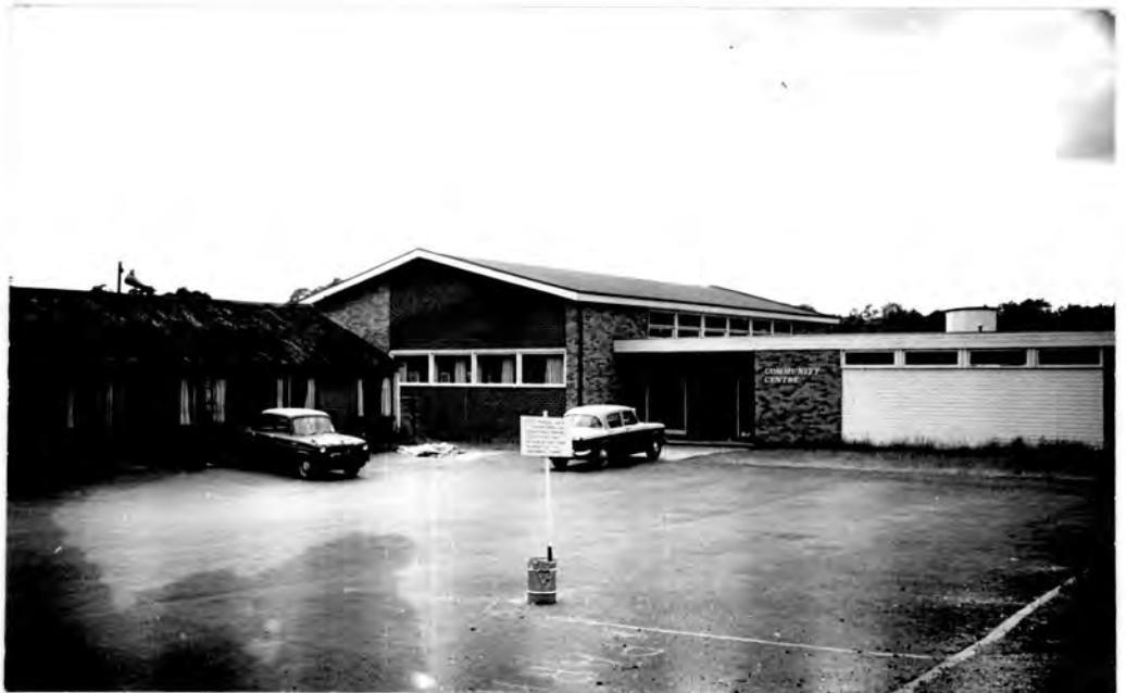
PLATE 57. The Community Centre, Devonshire Avenue. On the left is the original temporary building.
