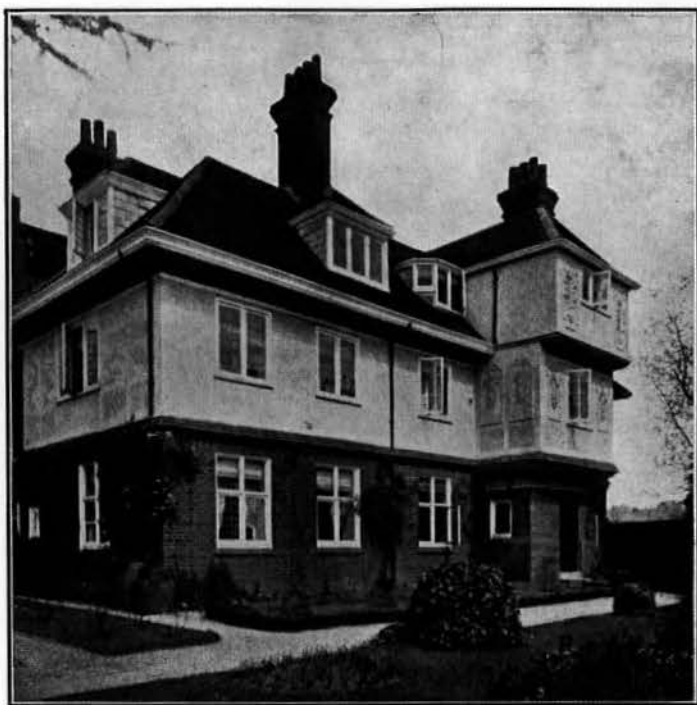
MASTER'S HOUSE AND DORMITORIES 1910
