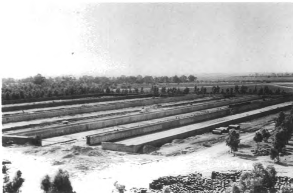
Plate 5.6. El Gwarsha Sewage Purification Plant (under construction, 1967)
