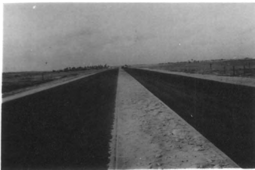
Plate 11.6. The new dual-carriageway.
