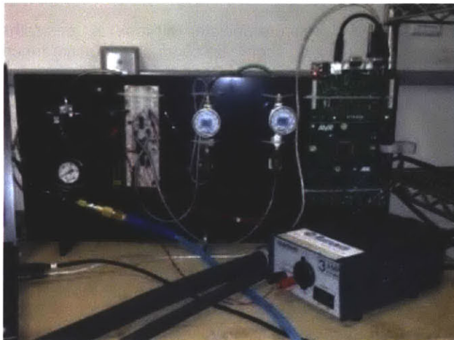
Figure 4.27 – Pneumatic control system and hardware.
