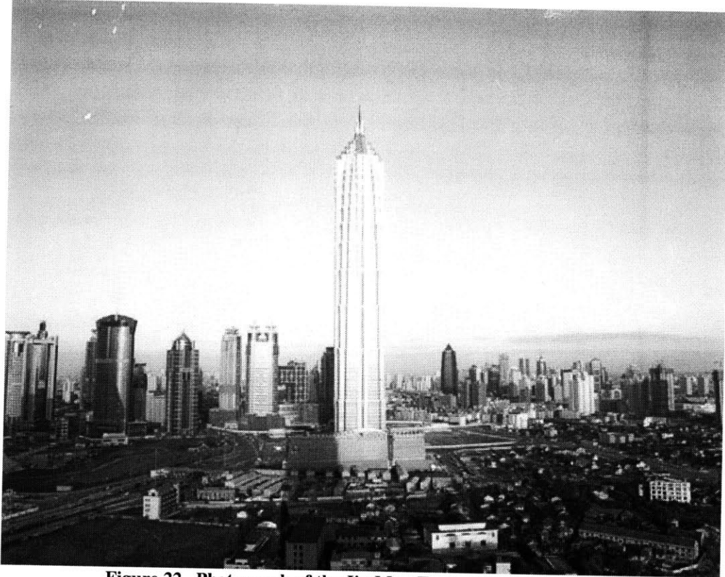
Figure 22. Photograph of the Jin Mao Tower (Shanghai, 2003).
