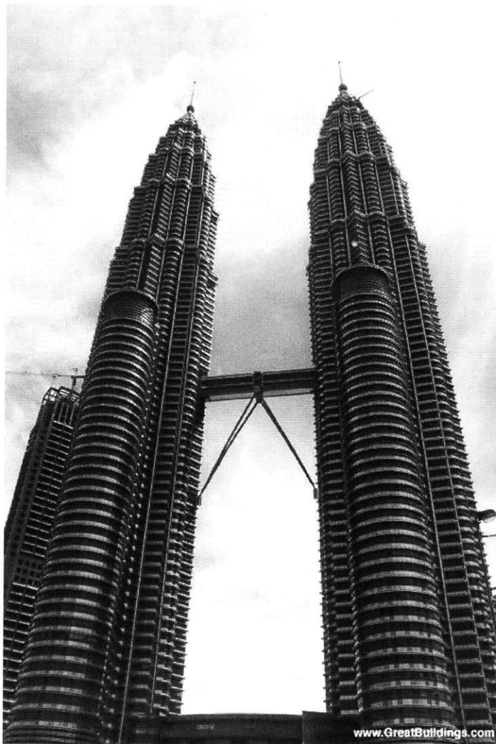
Figure 21. Photograph of Petronas Towers (Bocaling, 2000).
