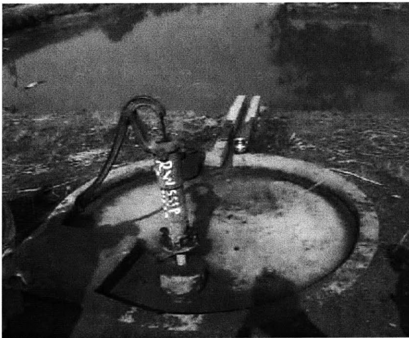
Figure 2 A Typical Suction Tubewell
