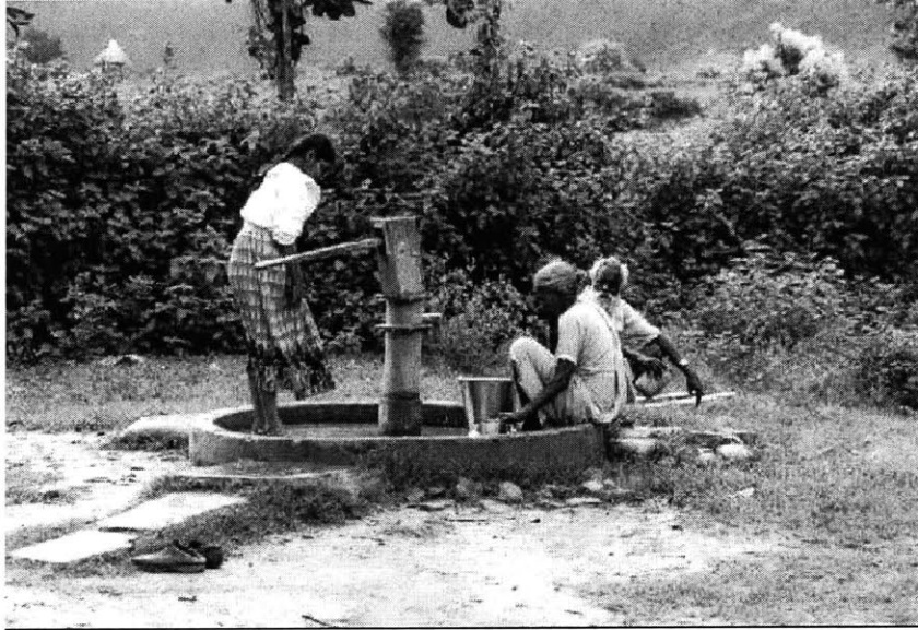
Figure 1 A Typical Lift Tubewell
