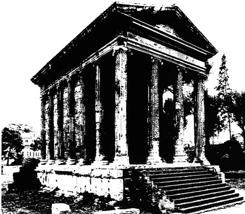
Figure 2-51. Rome, Boario Forum, temple of Fortuna Virilis, also called the Rectangular Temple (70 BC).
