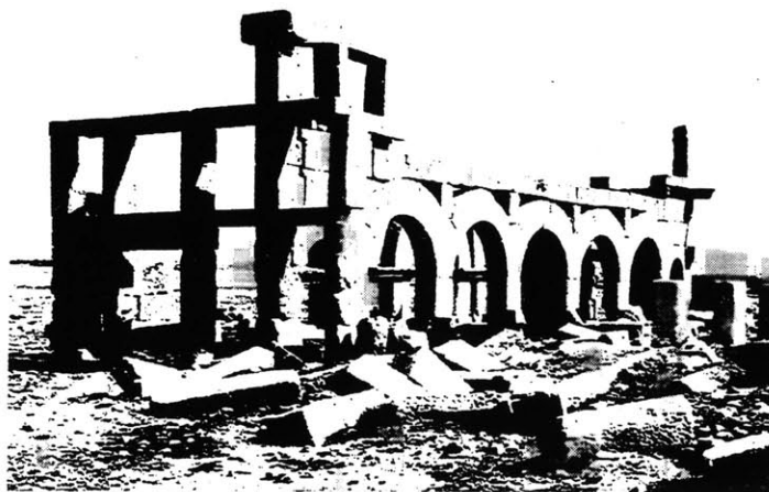
Figure 2-64. Brisagane (near Tébessa), oil production building.
