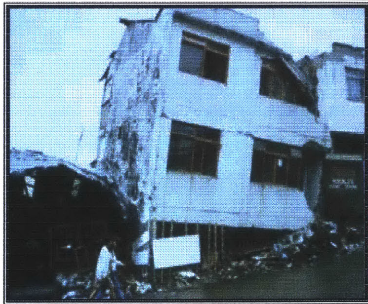
Figure 2.7 – Collapsed unreinforced masonry buildings in Colombia, after the earthquake of Armenia and Pereira on January 25 th , 1999.
