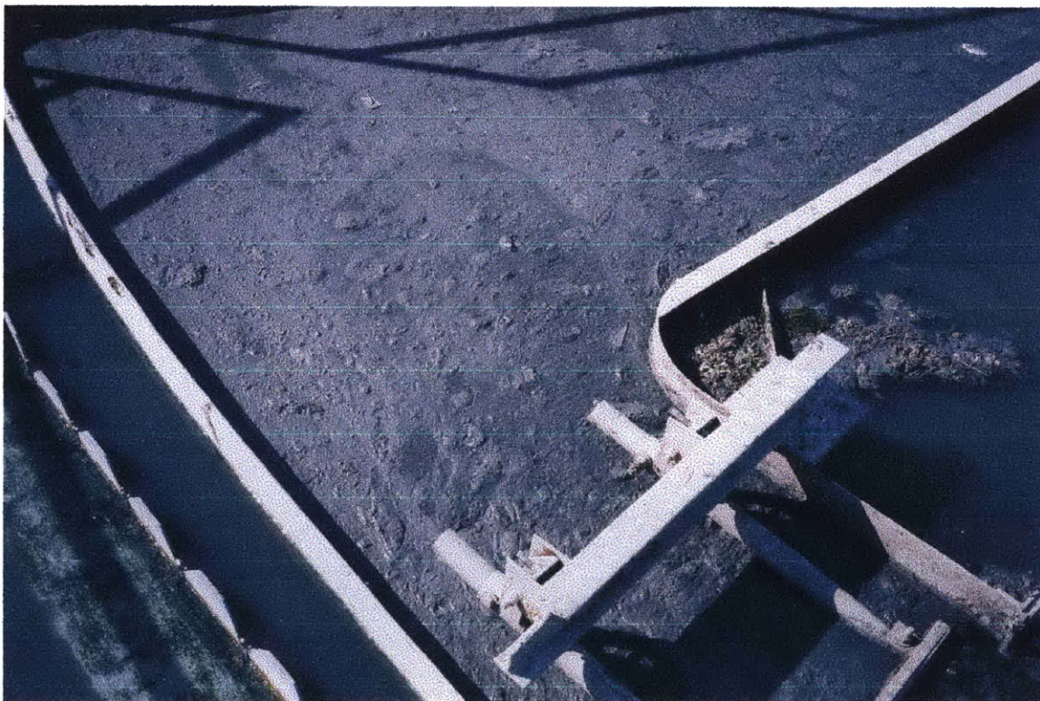
Figure 6: Floating sludge at Vega Baja
