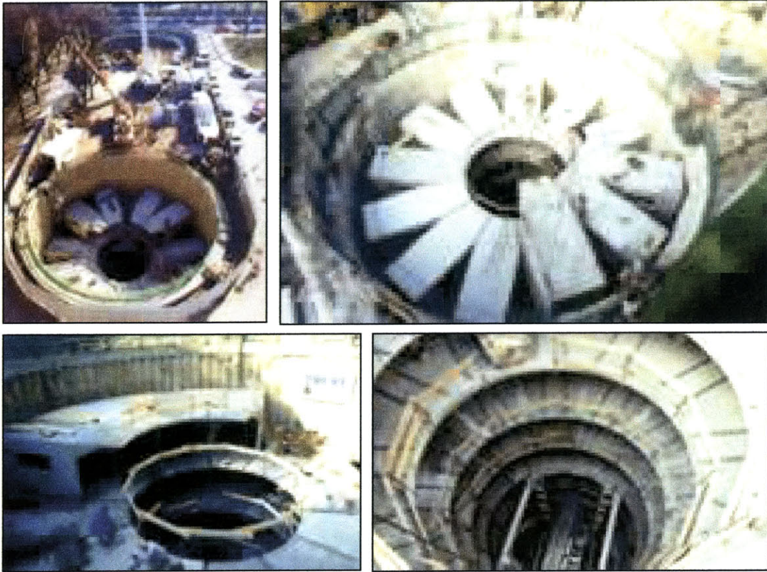
Figure 5.6 – Construction of a TreviPark
