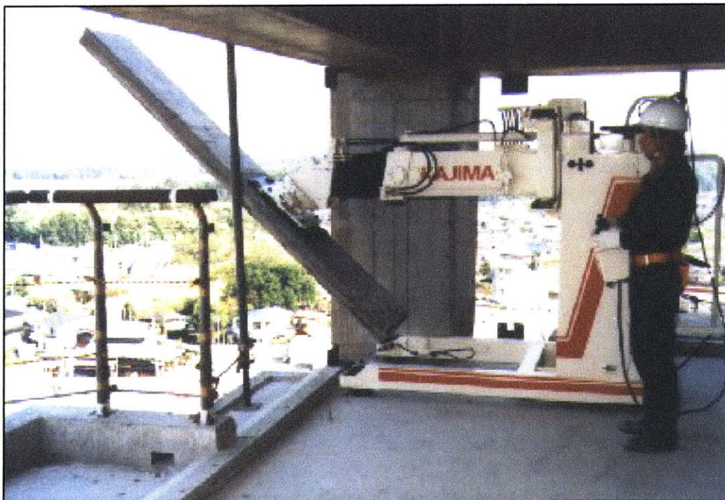
Figure 4.2 – Kajima Corporation, Board Placement
