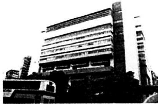
4. Kwun Chung Market in a high-rise multi-functional building for public services.
