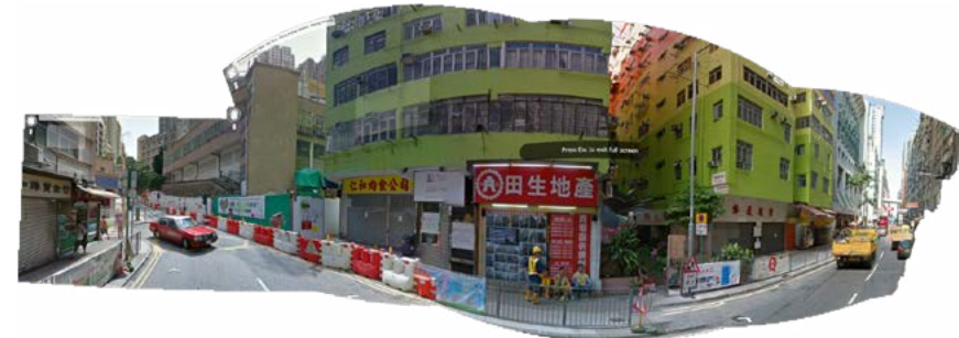
Figure 5.7 The Queen's Road West with the subway station in construction.
