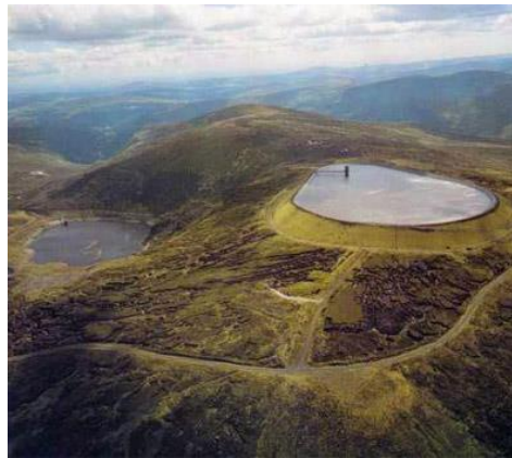
Figure 5 Turlough Hill pumped hydro power station Ireland [4].
