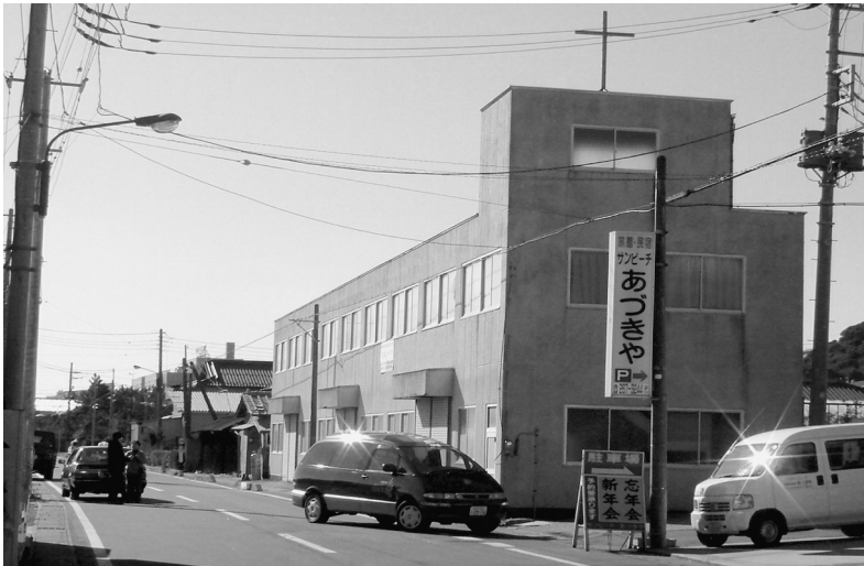
Picture 4: Rental building of the GMIJ since 2003 (Oarai, 2004).
