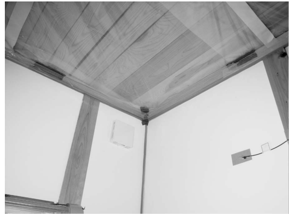
Figure 6. Sealing with Tape and sheet
