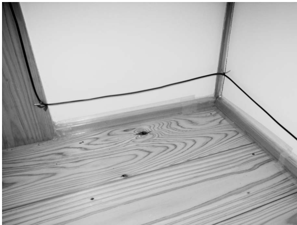
Figure 5. Taping on the end of floor
