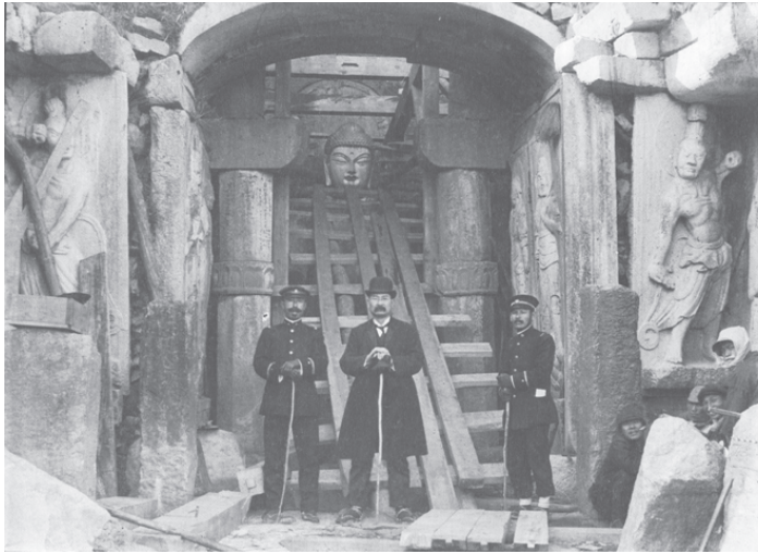
Fig. 6 Security guarding Sökkuram cave during reconstruction, Kyōngju (circa 1913). Note the wooden beams supporting the cave temple and Buddha. The photographer is identified as Mr. Tanaka from Tōyō-ken Studio. Source: Kim Tae-shik et al. Kyōngju Silla yujōk ūi ōche wa onūl: Sökkuram, Pulguksa, Namsan (Exhibition Catalogue of Glass Plate Photographs of Silla Remains in Kyōngju) Vol. 2, Seoul: Sōngyunkwan University Museum.
