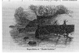
Rope-dikes, or "Snake-baskets". 繩の堤防, すなわち"蛇駕籠"
