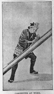
Carpenter at work. 仕事中の大工
