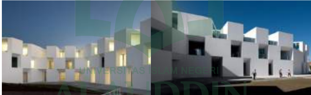
Gambar II.36 Fasade Residencias Assistdas
