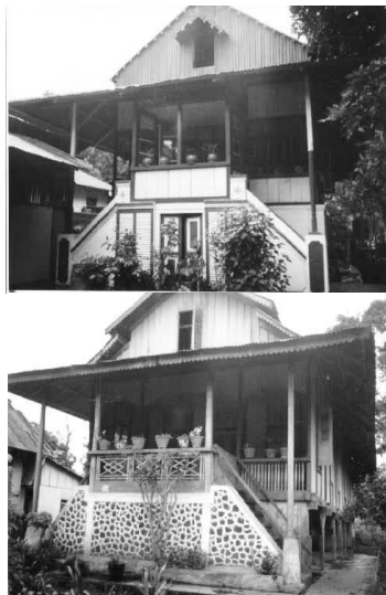
Fig. 5 Raised platform type of RTM with additional plane covering 'empty space' under the front stairs
