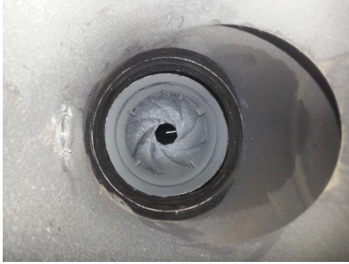
Figure 3-17. Orifice plate
