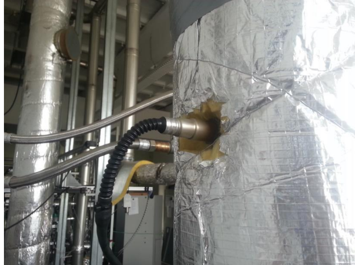
Figure 3-16. Lambda probe
