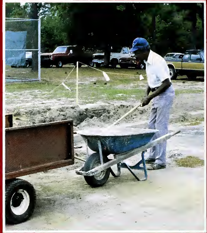
Construction workers rush to complete the new addition to Williams-Brice.
