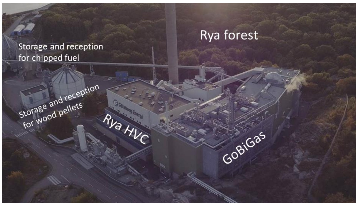
Figure 2.2: The GoBiGas plant (green building) and surroundings including the protected Rya forest.
