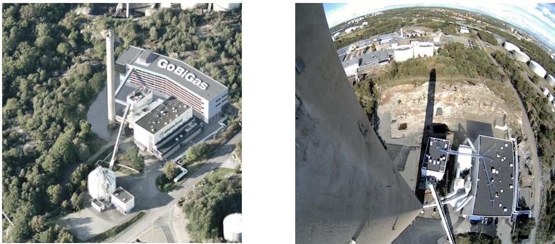
Figure 2.1: Photomontage of the GoBiGas plant from the planning phase of the project (left) located tight next to an existing boiler and the protected Rya forest, and picture from the site preparation.
