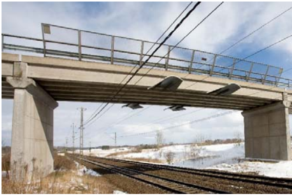
Figure 2: Concrete beam bridge investigated (source: NCC).
